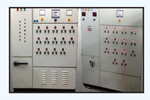
Capacitor Control Panels are provided for Controlling the Power factor of the Complete installation. The Front of the fully compartmentalized feeder for controlling Individual capacitors. Whereas rear side of the CCP House Individual capacitors. Whereas rear side of the CCP House
